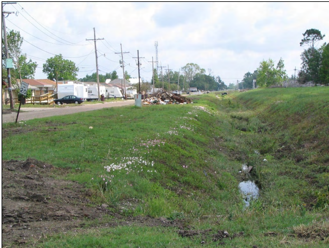
Photo 3. Typical Roadside Ditch Collector
