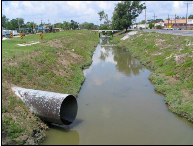
Photos 4 and 5. Storm Sewer Outfalls into Canals
