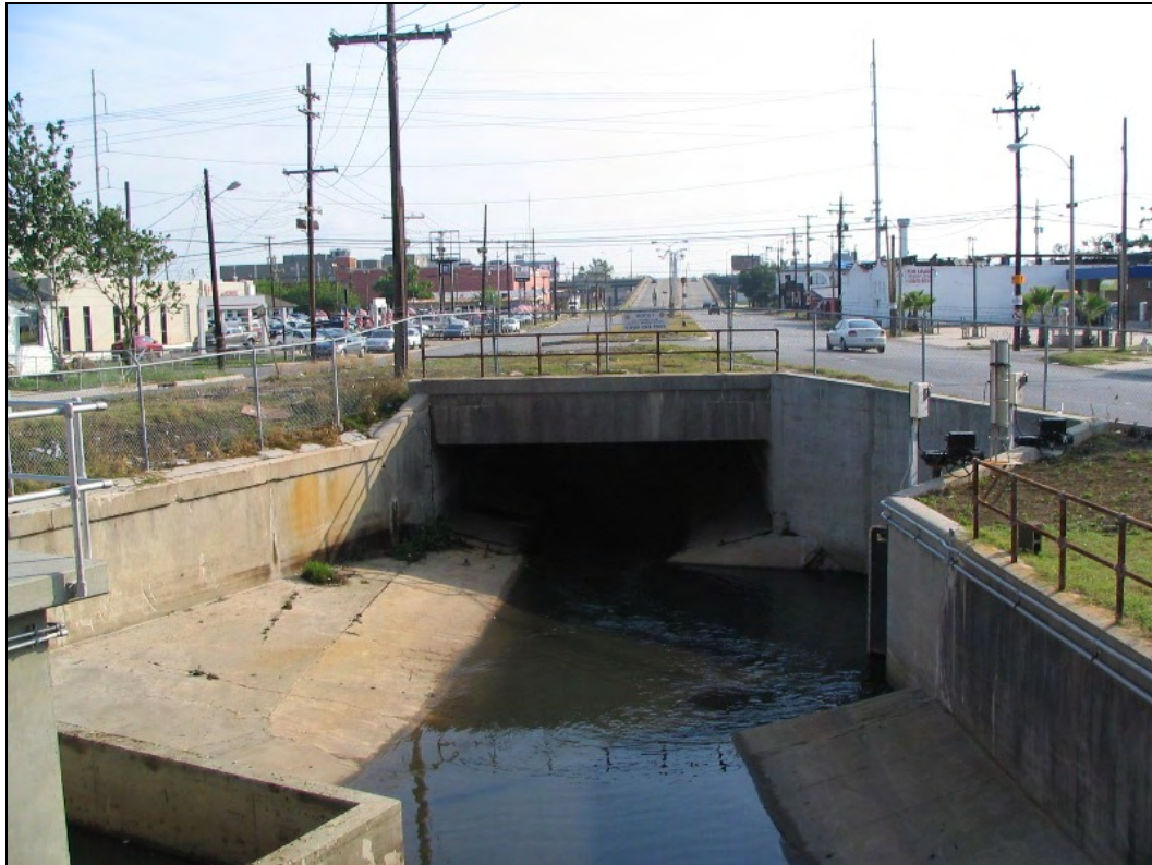
Photo 3. Broad Street Canal Entering Pump Station #1
