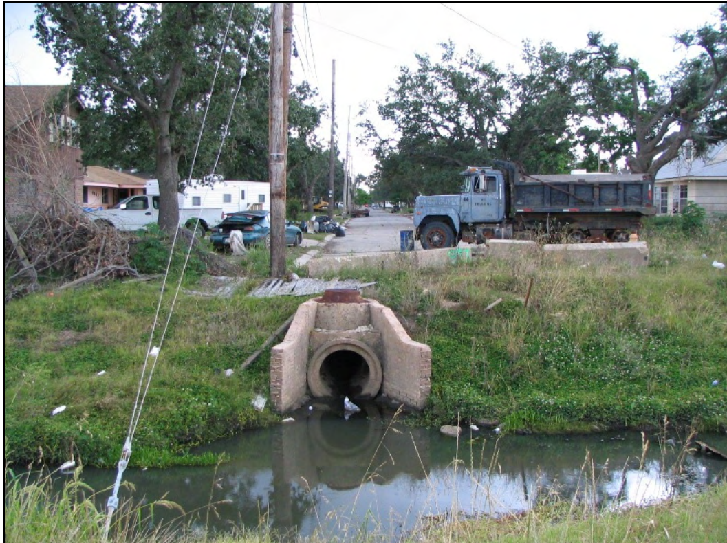
Photo 3. Storm Sewer Outfall into Dwyer Canal
